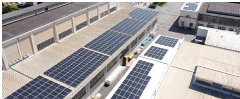
of 961 photovoltaic modules were initially installed – which is equivalent to an area covering 1,634 m<sup>2</sup> – on the roofs of the office and production buildings at its Austrian facility. 43% of the power that Bekum uses every
